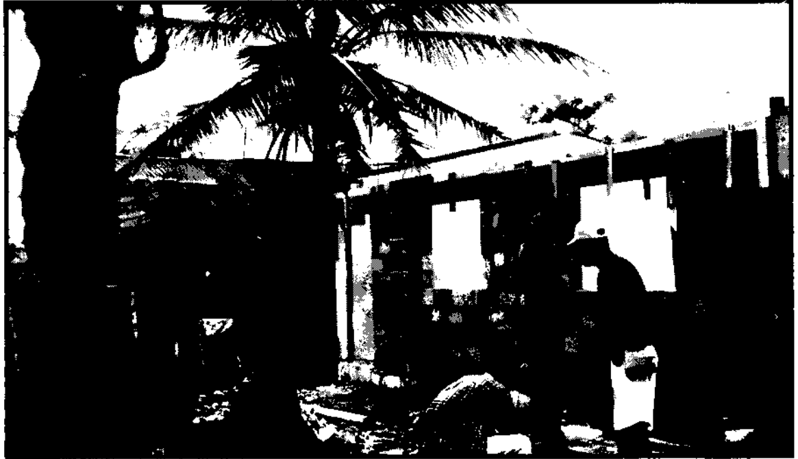
Residents of the community are rebuilding the school in Batey Altogracia.
